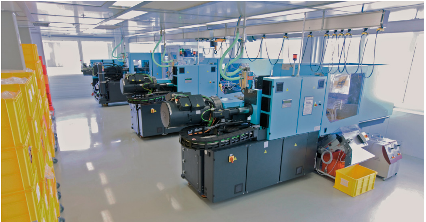
In SLG's clean-room, two all-electric IntElect machines (at the front) and an El-Exis hybrid high performance machine of Sumitomo (SHI) Demag are now used for production purposes.
