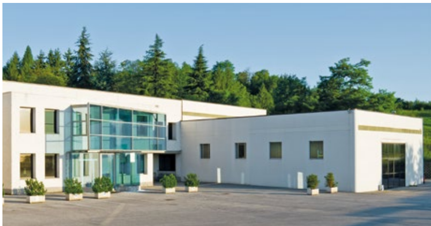
In an area of approximately 9,000 square metres, Electro-Parts produces linear actuators, gear motors, PMDC motors, electric fans as well as brushless motors
